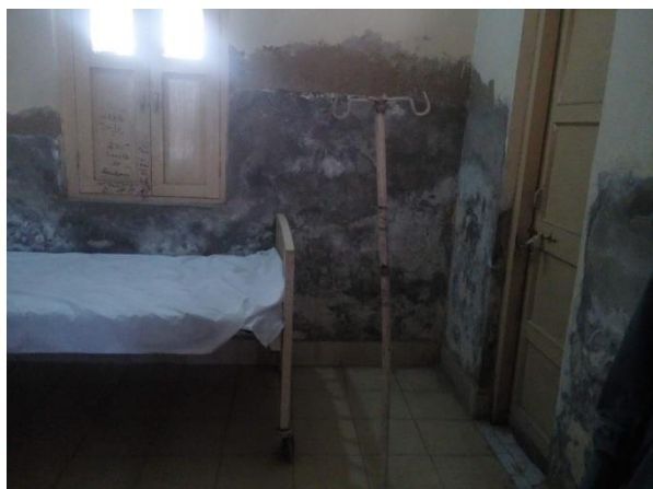
Figure 1. 1 Emergency room in RHC facility, Kashmore
